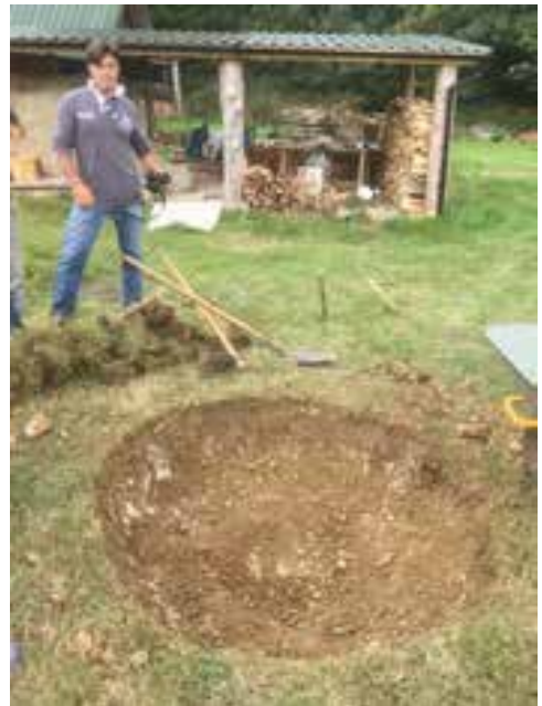
Robin Wilson with the finished pit
